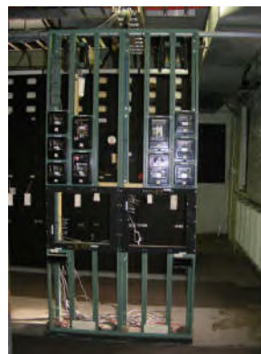
Fig. 1. Examples of Electromechanical Relays Installed on Relay racks
