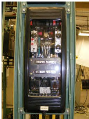
Fig. 1. Examples of Electromechanical Relays Installed on Relay racks
